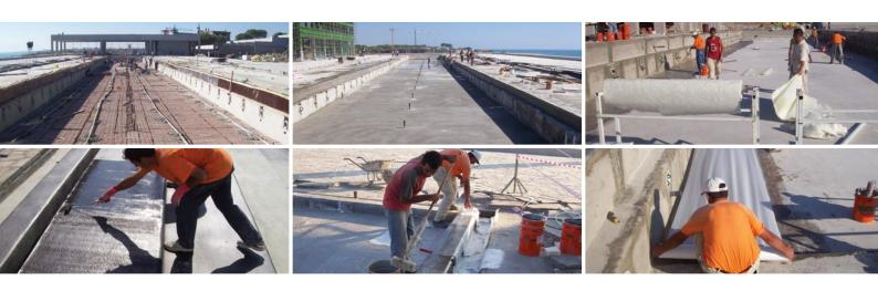
The pool surfaces were laminated with CSM, and then METYX Composites peel plies were used to prepare the surfaces for the secondary operation, which was an epoxy base coat followed by a polyurethane coating finish. We were able to supply a large quantity of peel plies with very short
